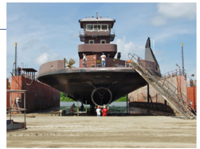
CLICK HERE to follow the progress of the TxDOT ferry.
