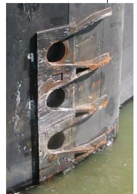
Pin receptor post modification to a barge.
